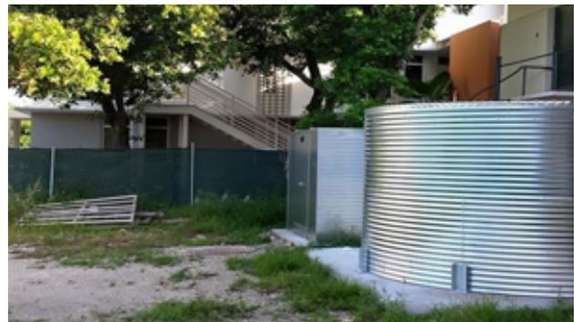
On the RSMAS campus, a closed loop system has been installed in the Chiller plant: 90% of condensate water is recirculated in the system as makeup water for the cooling towers. Submeters have been installed to measure the percentage of condensate in the mix, generating an average of 300 gallons per day or 10% of the cooling tower demand.
